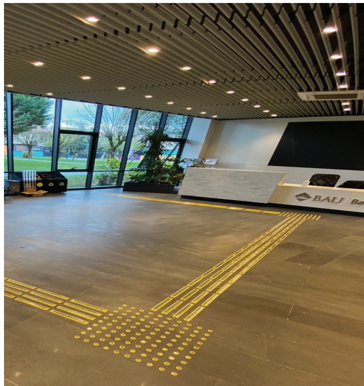
Photo 1: A sensible guide road prepared for disabled people in Kemerburgaz Campus
